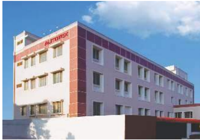
Autotex Corporate Office - Unit I
